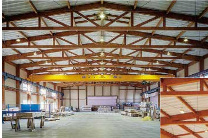
Truss (structure) can be found in a number of buildings. JKHD Group's KEYTEC plant is a truss structure.
